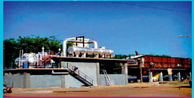
Nuclear Desalination Demonstration Plant Kalpakkam
