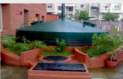
Nisargruna at Symbiosis University, Pune to process waste food from the canteens
